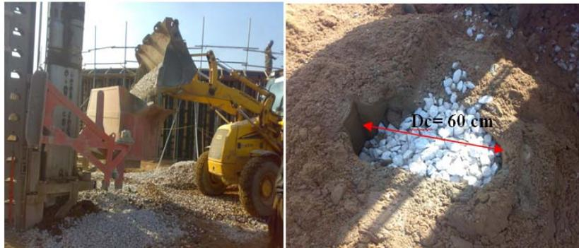
Figure (1): Installation of stone columns
