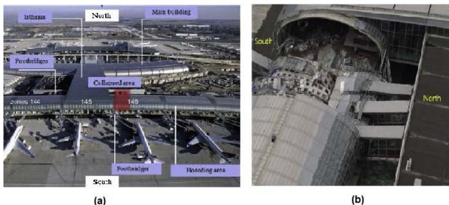
Figure (1): (a) View of the terminal and (b) Collapsed area of the terminal (El Kamari et al., 2015)
