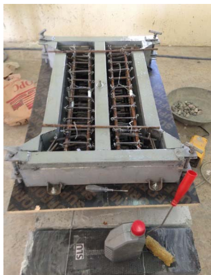
Plate (2): Steel molds and reinforcement cage
