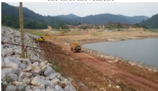
Figure (4): Rehabilitation work after first failure
