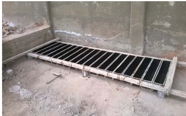
Figure (2): Formwork of columns with fair face panels
