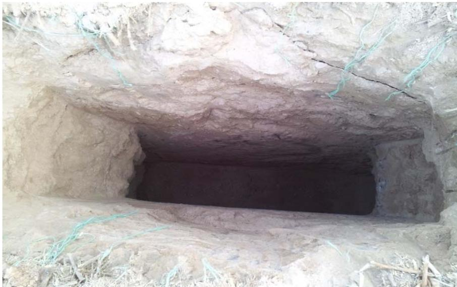
**Figure (6):** Excavation below ground surface was made to a maximum depth of 2.5 m using a backhole at the studied sites
