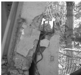
**Figure (1): Failure due to insufficient splice length at the top and bottom of the RC column in Bingöl (Turkey) earthquake, 2003 (NISEE)**
