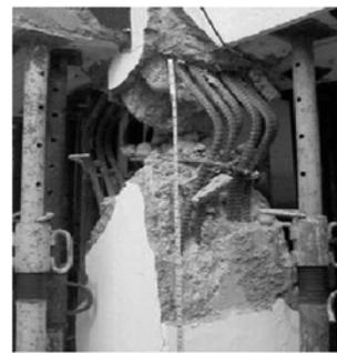
**Figure (2): Severe damage in the RC column due to widely spaced transverse reinforcements in Columbia earthquake, 1999 (NISEE)**
