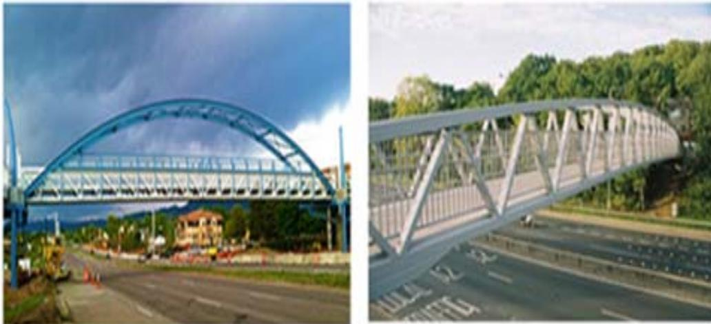
Figure (1): Truss footbridges
