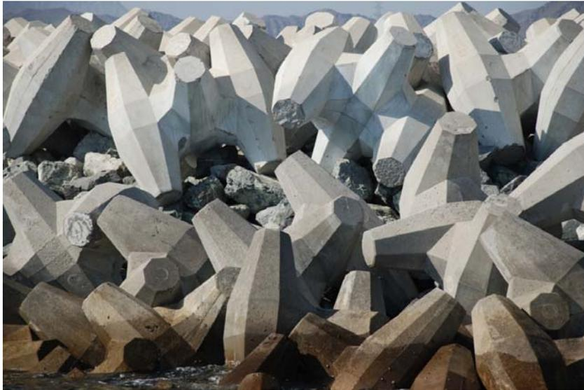
**Figure (4): Movements of concrete armour units with large settlements [Source: Hendrikse, 2014]**
