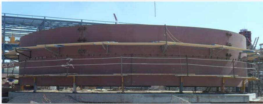
Photo (1): Construction of the water tank
