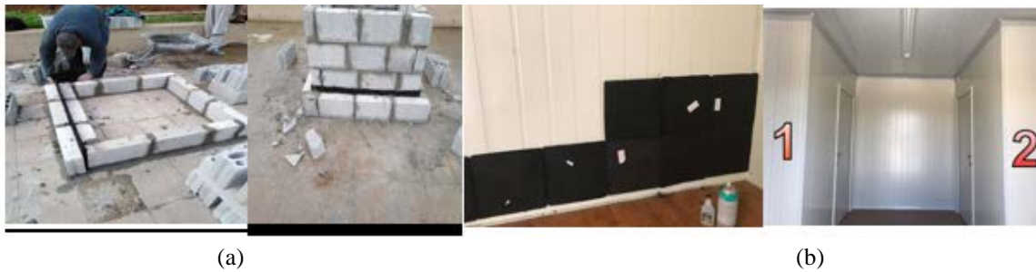
Figure (1): a) Construction of two rooms built from bricks b) Construction of two caravan rooms made from rigid polymer
