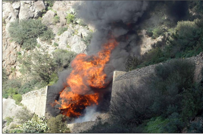
Figure (1): The fire of El Akhdaria Tunnel (Algeria)
