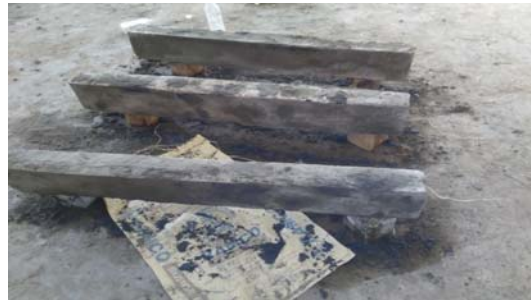
Figure (3): Repaired beams
