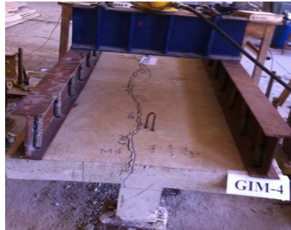
Figure (15): Crack pattern in the slab of specimen GIM-4
