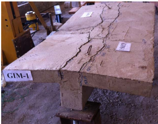
Figure (12): Crack pattern in the slab of specimen GIM-1
