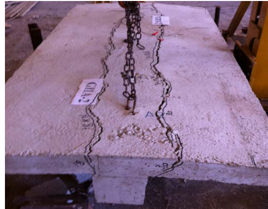
Figure (18): Crack pattern in the slab of specimen GIIA-2
