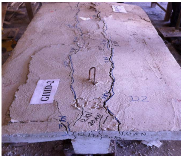
Figure (20): Crack pattern in the slab of specimen GIID-2
