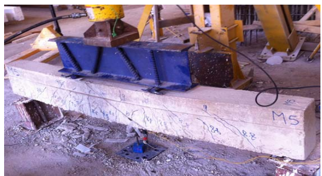
Figure (16) (a): Crack pattern in the beam of specimen GIM-5
