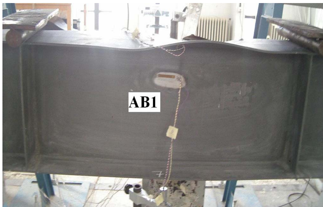
Figure (10): Local Buckling Mode in Beam AB1.
