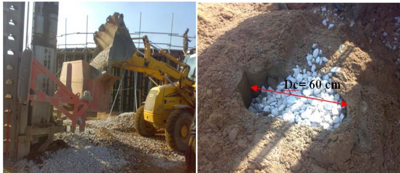
Figure (1): Installation of stone columns
