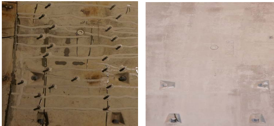
(a) Image before treatment (b) Image after treatment Figure (11): Comparison shots before and after treatment
