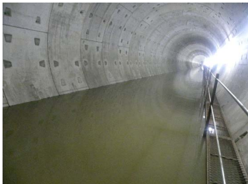
Figure (3): Scene photos of tunnel water gushing
