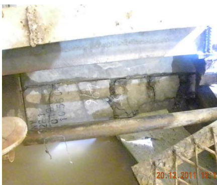
Figure (3): Scene photos of tunnel water gushing
