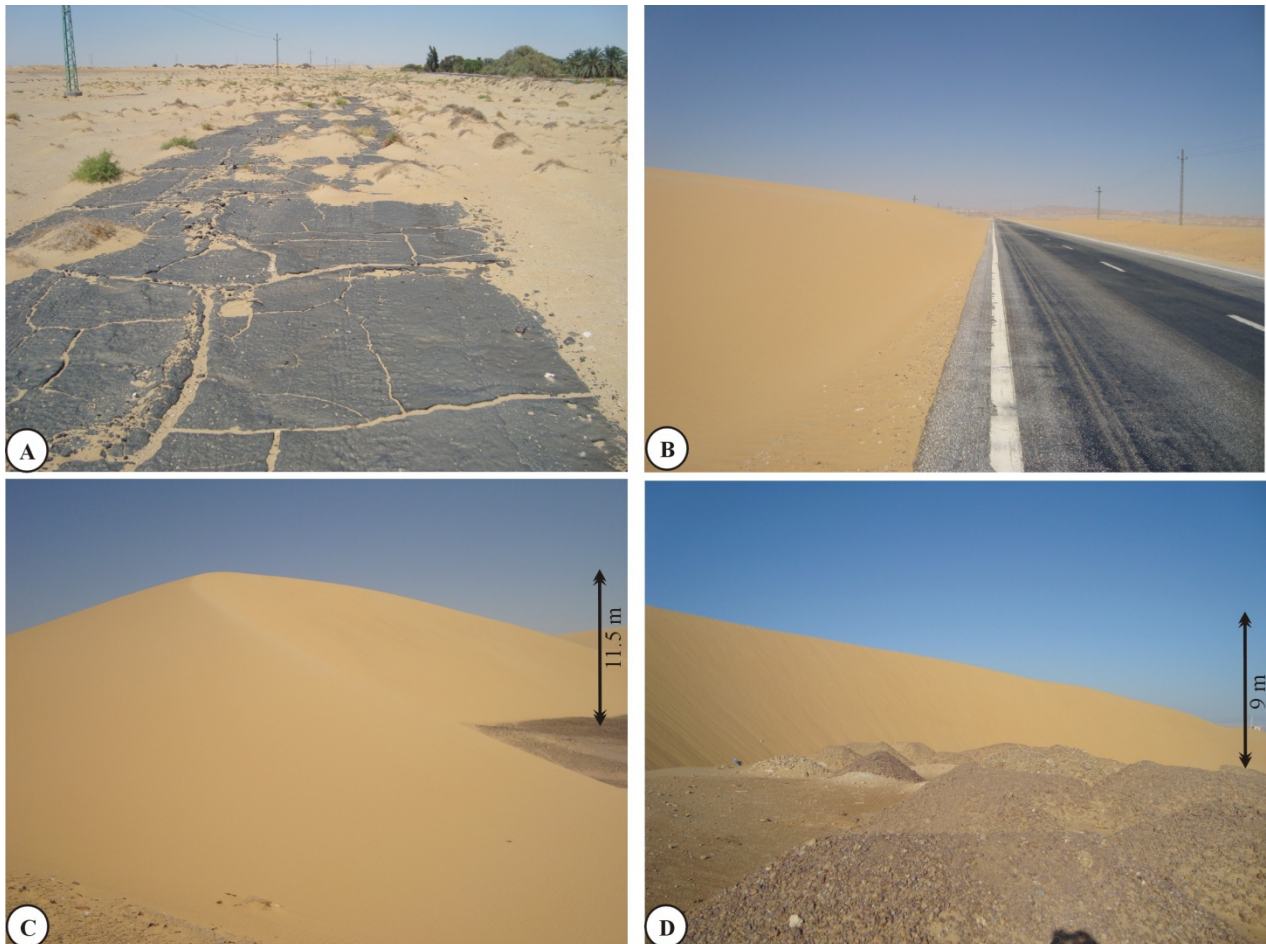
Figure 2: Field photographs of sand dunes showing; (A): destructive effect of sand dunes along old Kharga-Assuit asphaltic road; (B): destructive effect of sand dunes along present Kharga-Assuit asphaltic road; (C): barchan sand dune to the east of El-Bagawat Cemetery (site II); and (D): barchan sand dune along Kharga-Dakhla asphaltic road (site III)
