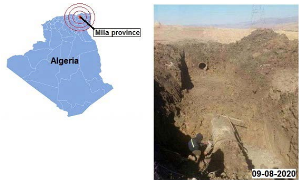
Figure (2): The 7 th August 2020 earthquake effects: Pipeline repair operation
