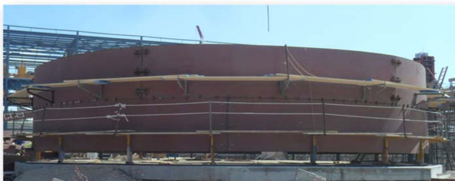
Photo (1): Construction of the water tank
