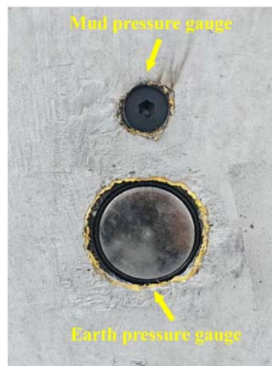
(b) Mud pressure gauge and earth pressure gauge installation
