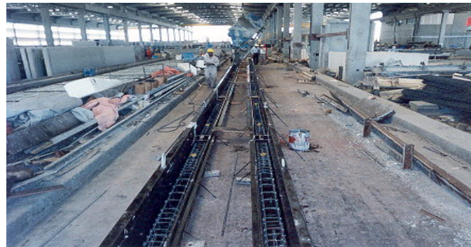
Figure 2: Fabrication of beams in the pre-stressing bed
