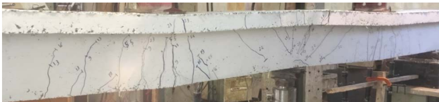
Figure (5): Typical failure pattern for beams S1, C1 and C2
