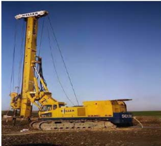
Figure 1: Mixing method with (a) on board binder silo; (b) separate binder silo
