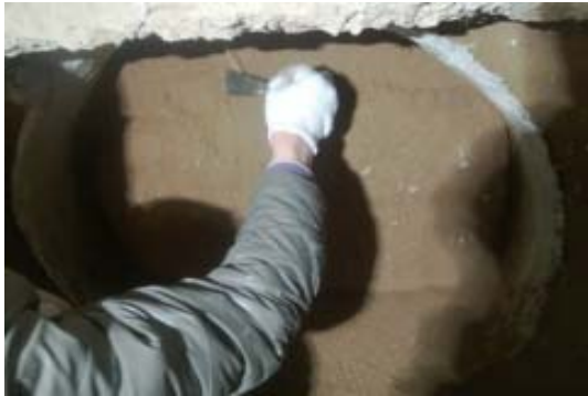
Figure (4): Excavation of soil
