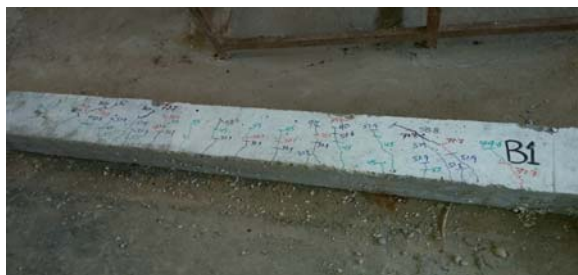
Figure (4): Control beam (B1) after failure
