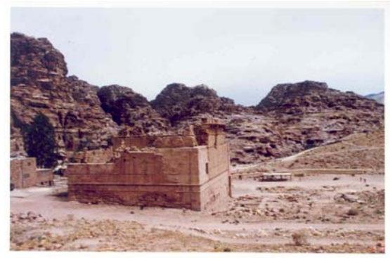
Figure (5): The lower part of the southern wall
