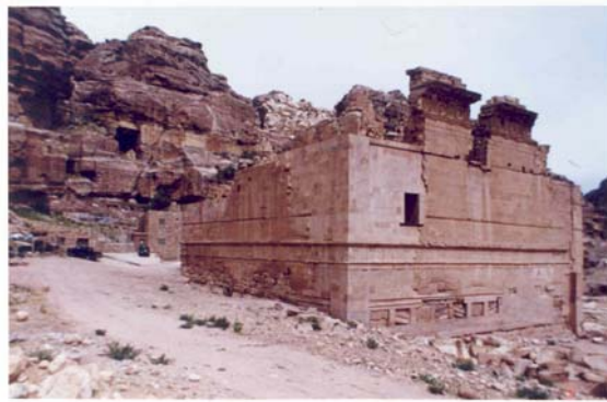
Figure (4): The south-eastern corner
