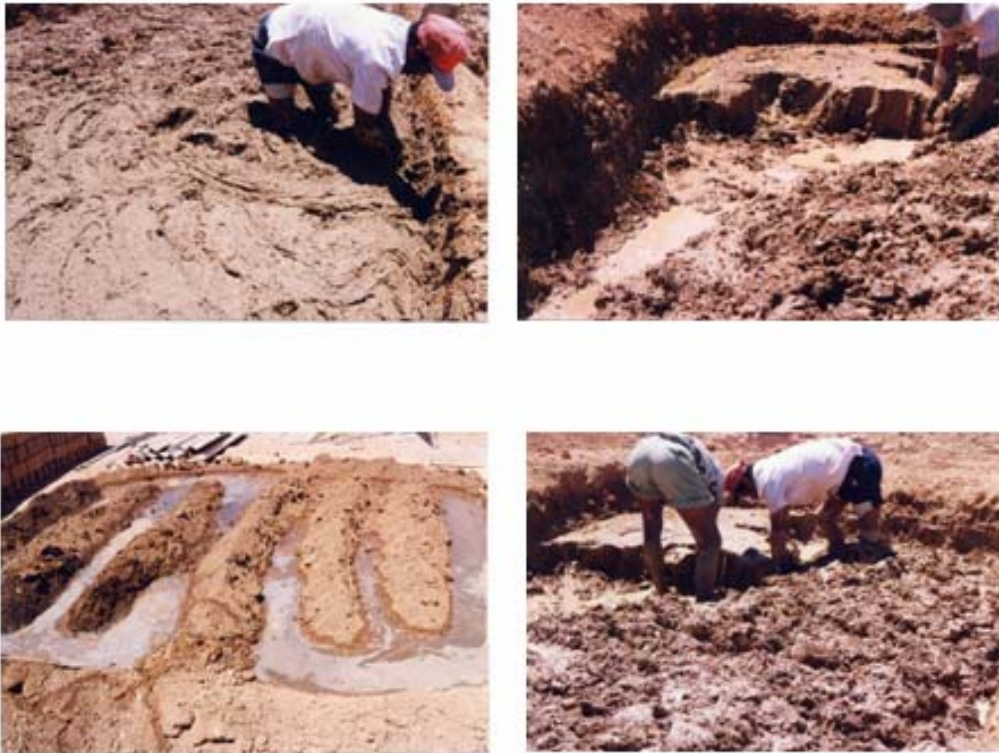
Figure 1: Mud mixing operation
