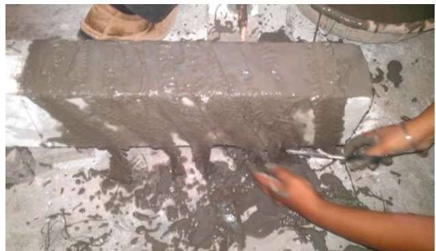
Figure (2): Wrapping with glass fiber strips and cement based composites
