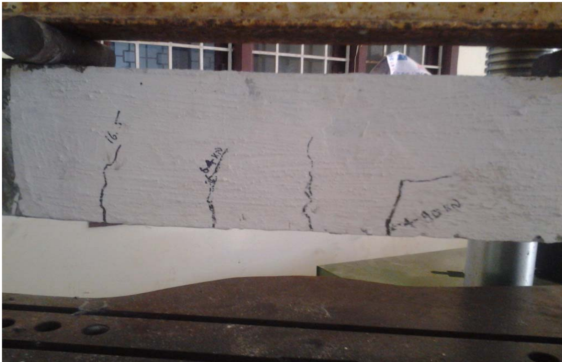
Figure (5): Initial flexural cracks in retrofitted damaged RSD beam
