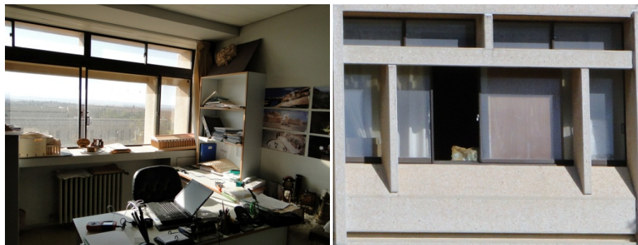
Figure (6): Office interior details (left) and window details from outside (right)
