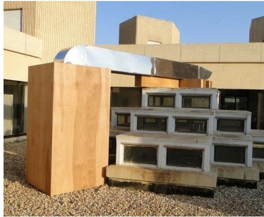
Figure (7): The actual anidolic duct and the experimental chamber
