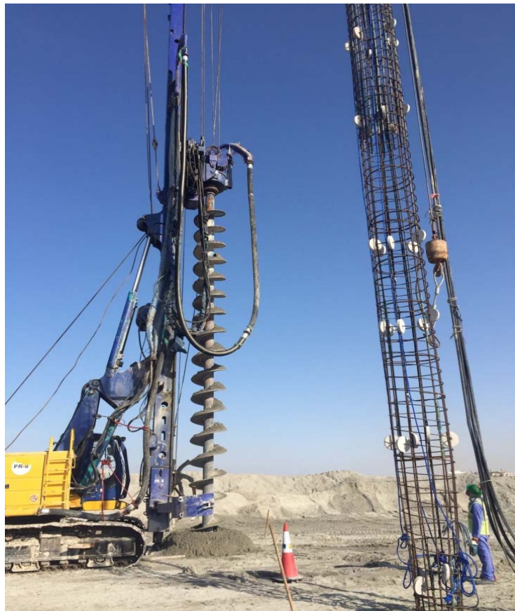
Picture (1): CFA pile installation
