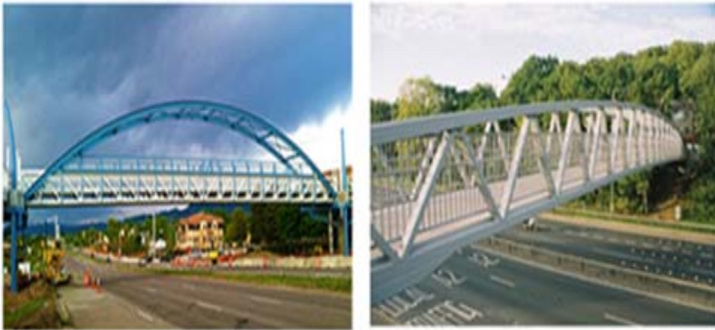
Figure (1): Truss footbridges
