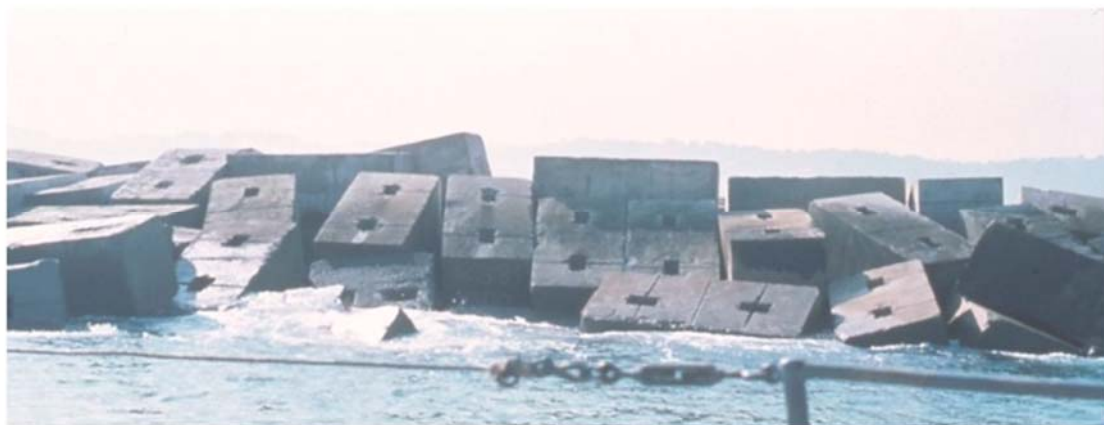
Figure (2): Breakwater armoured with rectangular blocks constructed in the 1930s [Source: (Jensen, n.d.)]
